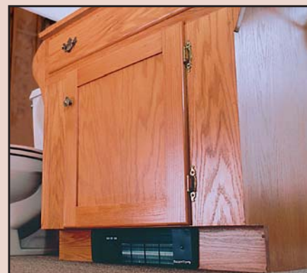
Twin-Flo III heater bathroom cabinet installation.
