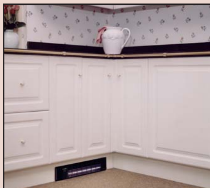
Twin-Flo III heater kitchen cabinet installation.
